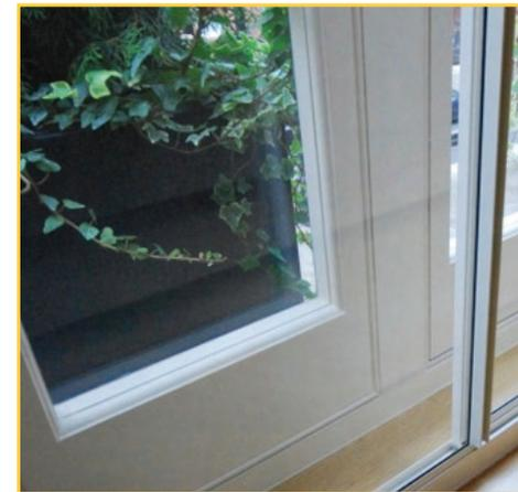
strong adhesive. This form of glazing can include sliding or hinged panels, enabling the windows behind the secondary glazing to be opened but is best left to a professional glazing installer.
